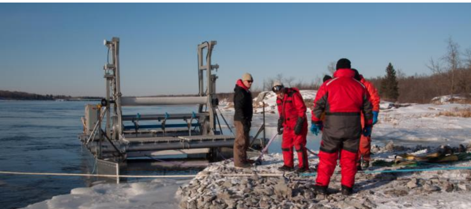
Turbine deployment on fast river in -20 deg conditions
